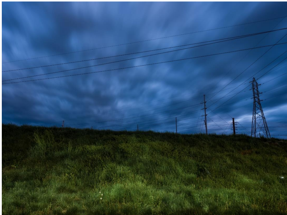
Figure 9: David Christian Rehor, Hidden Substation, Cook Drive, 2021. Pigment print, 16 in. x 20 in.
