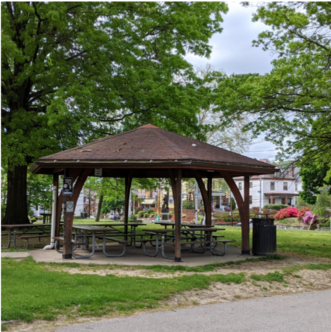
FIGURE 17. Pavilion at Bayne Park, Bellevue
